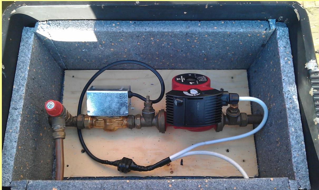
*The pump is positioned on the return with the PRV after the motorised valve.*
