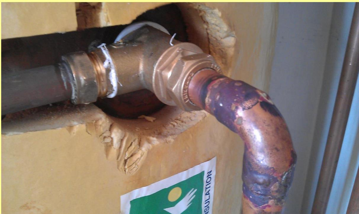
***This allows two entry points into one connection normally used on shower installations at the top of the cylinder.***
