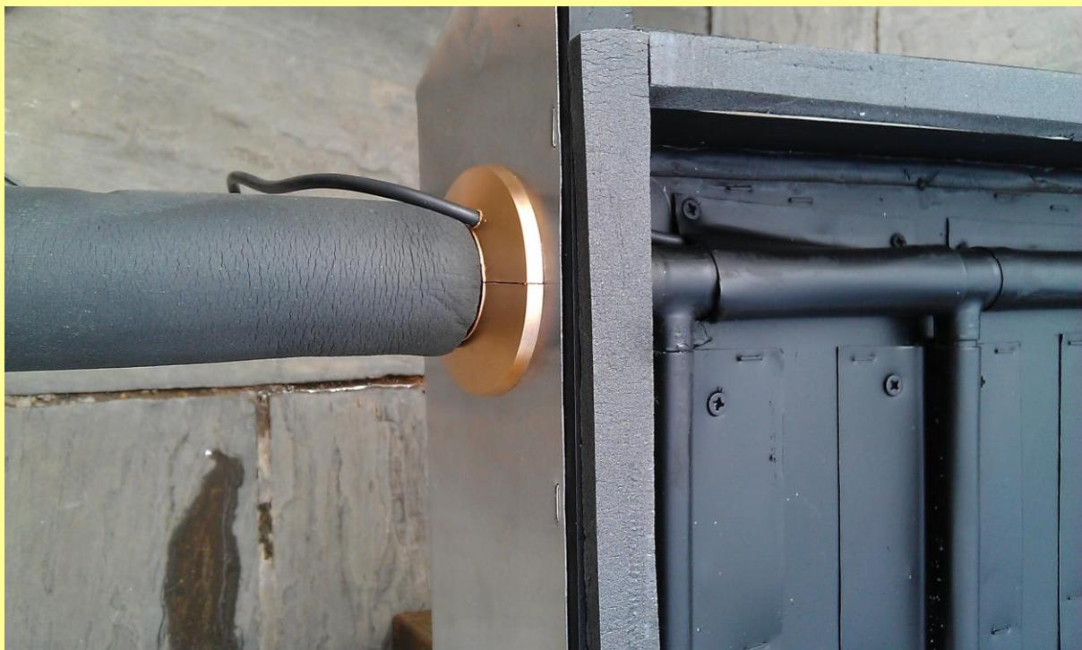
*The external pipe-work was insulated with 12mm thick armafex to stop heat loss.*
