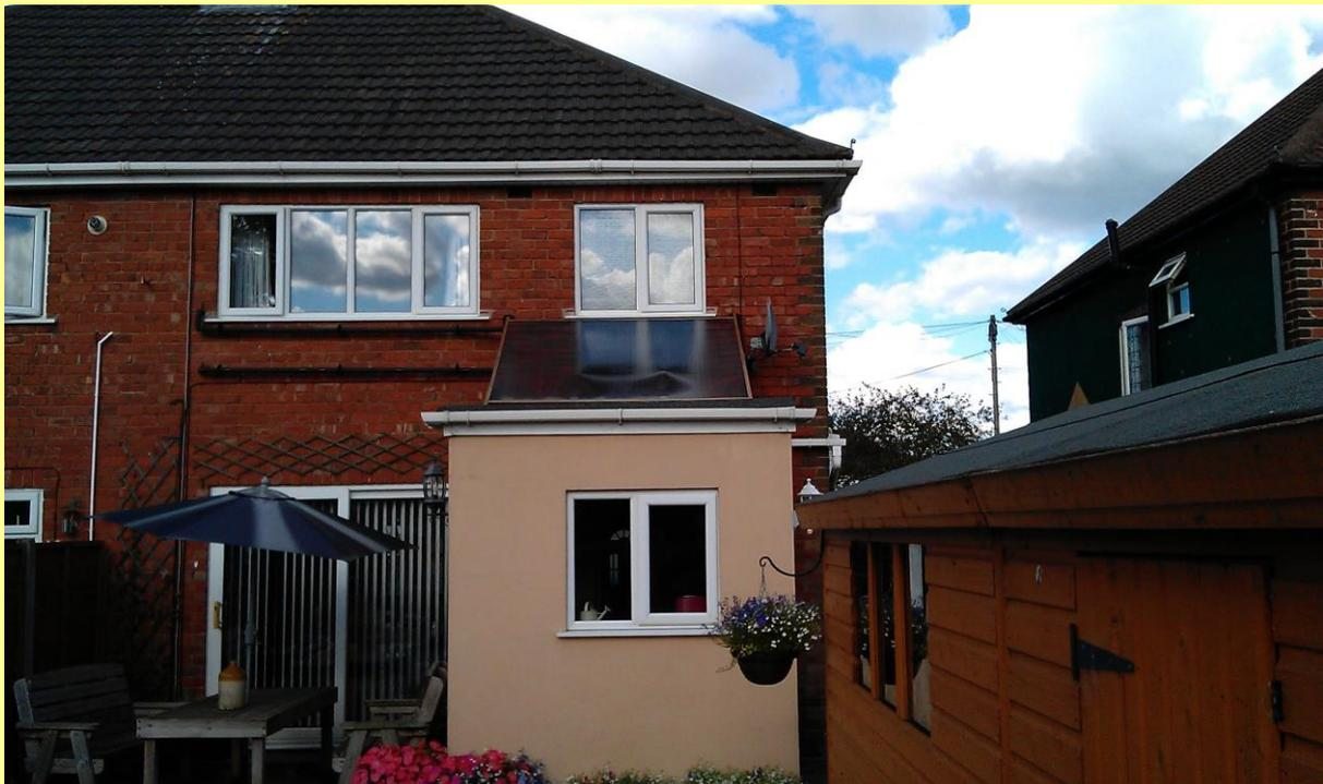
I started the panel by making my manifold out of 15 and 22mm copper pipe. I set the copper risers 135 mm apart. 15 of them. These connected to headers that were 22mm. I put a fall on the headers so it would drain down totally for the winter period.
