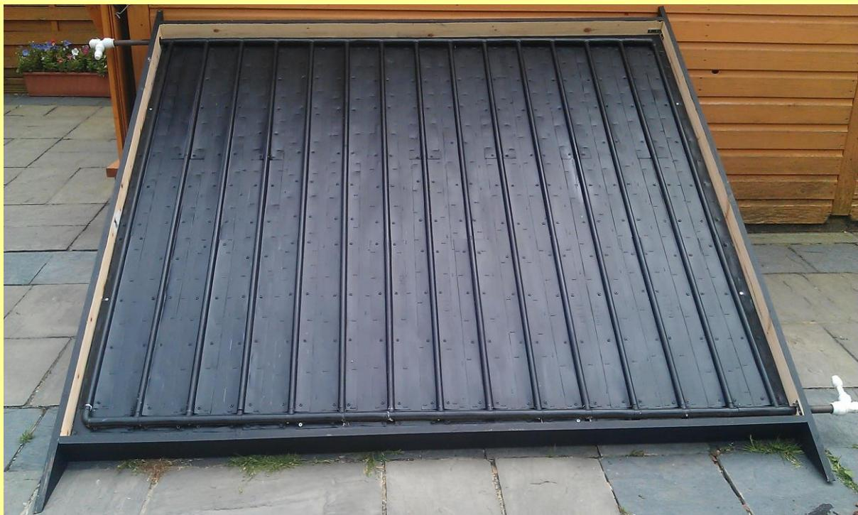
***The framework was designed to be self supporting. The framework was cut at the angle the panel was to be positioned at. I also waterproofed the framework before painting it with 3 coats of black exterior paint.***
