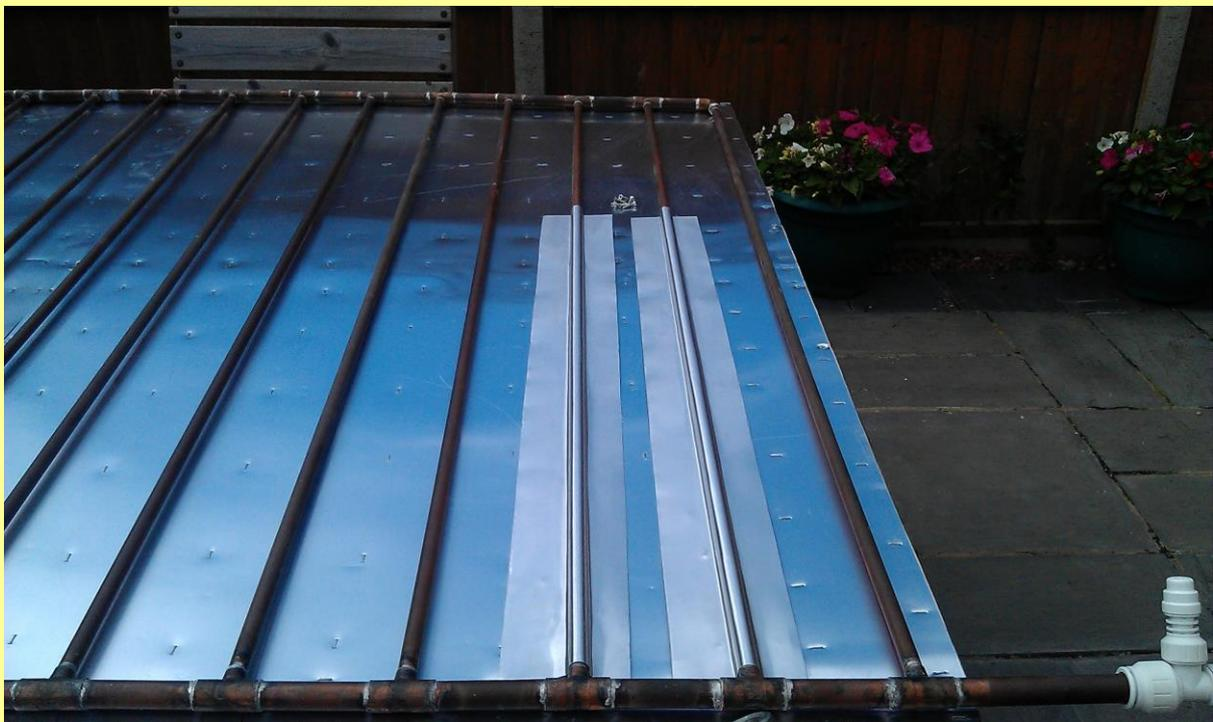
***I pressured tested the manifold at 5 Bar before covering with aluminium sheet.***
