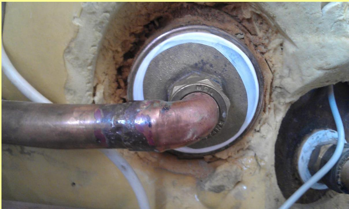
*I took out my immersion heater to incorporate a connection at the bottom of the cylinder. An immersion heater in a thermal store is used as a back-up heat source if the boiler breaks down. There about as good as a chocolate tea-pot on this cylinder.*
