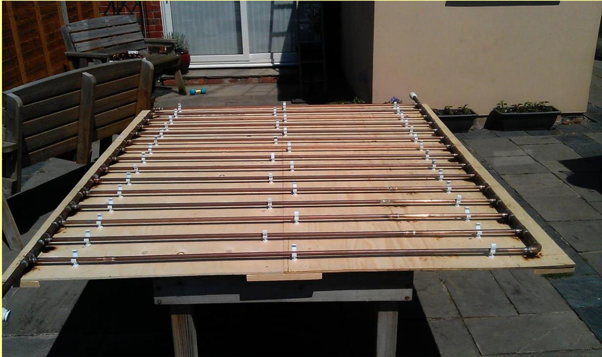
***The pipe clips are only there to aid make the manifold. Note the fall to the bottom of the panel.***
