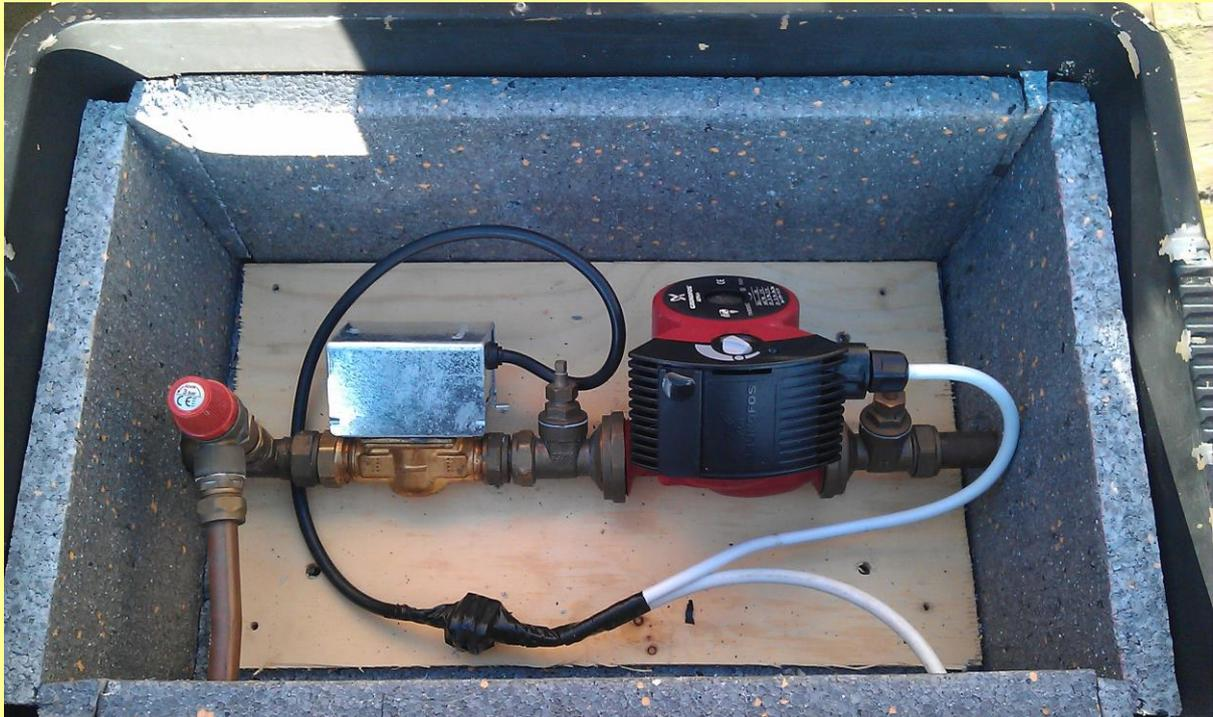
***The pump is positioned on the return with the PRV after the motorised valve.***
