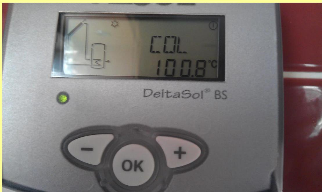
***I turned the controller on in winter (the panel was decommissioned) when we had a sunny day to see the temperature in the panel at 100.8°C. The outside air temperature was 7°C.***
