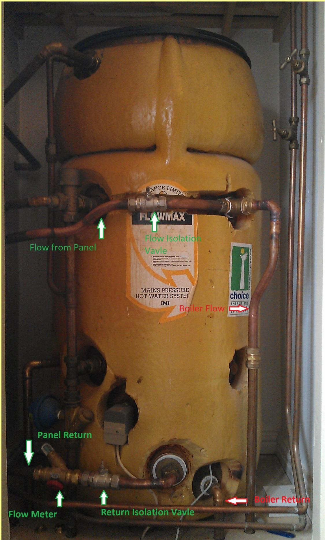
The space inside my airing cupboard is very limited and as you can see from the photo the isolation valves do not have any levers on them this is because the door will not shut if left on so they have been removed. It is also good because nobody can accidentally turn them off or temper with them, so a bonus in some ways.
